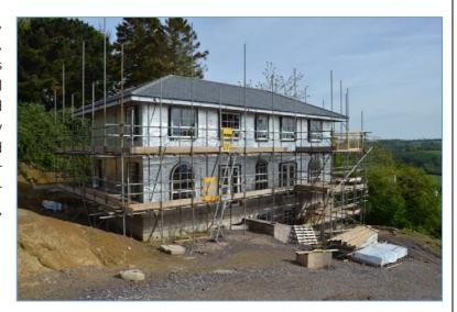
Unit 2 — 4 bedroom detached dwelling, roof structure complete but only part slated, no external windows and doors fitted, internally joists and studwork but no finishing, some first fix complete.
