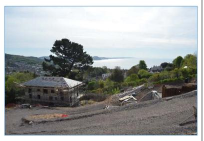
Unit 3 — 4 bedroom detached dwelling at early stage of construction, block and beam floors in at DPC level and some retaining piling/walling in situ.
