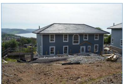
Unit 5 — 4 bedroom detached dwelling, roof complete and slated, external windows and doors in place, partly externally clad, internally chipboard flooring installed, walls plastered, first fix electrics and plumbing, kitchen/utility part installed.
